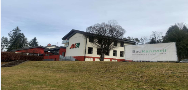
Conference venue before works | Source: BauKarussell
