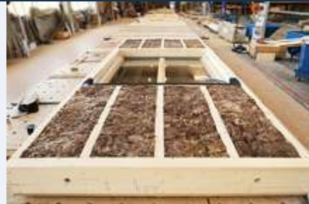
Prefabrication of façade modules | Source: Klimafond/Krobath
