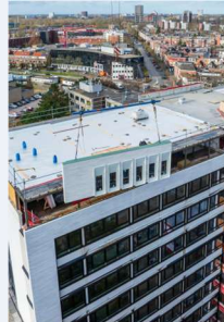
Prefabricated façade module hoisted into place | Source: WEBO
