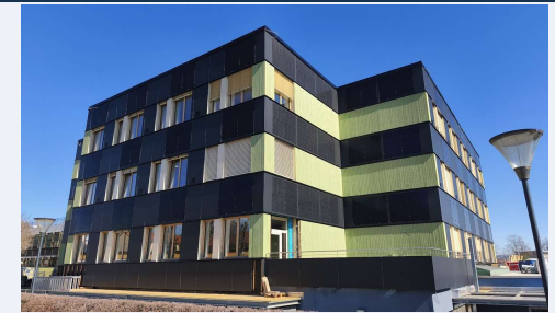
Renovated façade | Source: AEE INTEC
