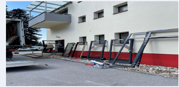
Recovered door-frame components | Source: BauKarussell
