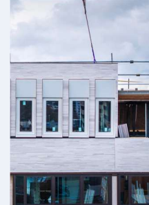
Renovated façade installation | Source: WEBO
