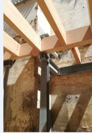
CLT beams on steel frame, detail | Source: ACR
