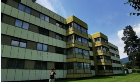
Before renovation | Source: AEE INTEC
