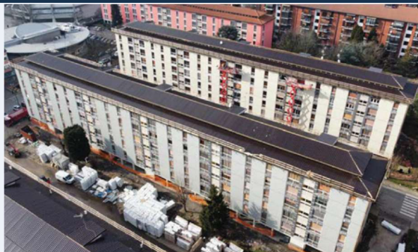
During renovation | Source: EDERA and Isopan
