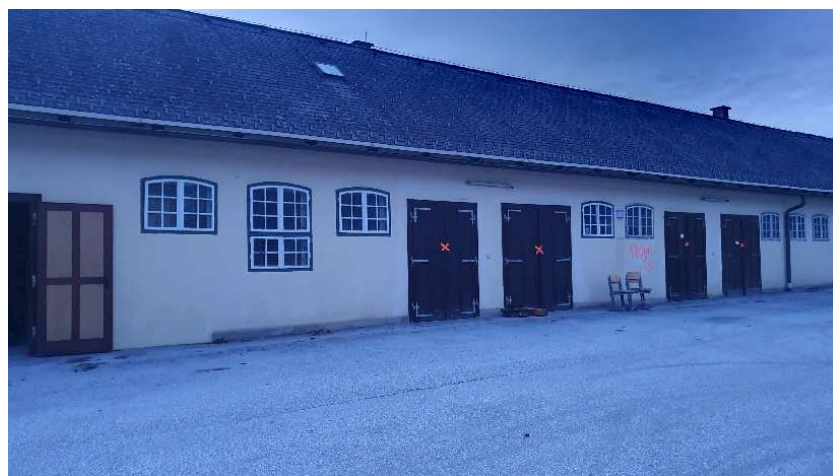
Figure 55: Safety precautions for Nogo areas for site visitors © BauKarussell
