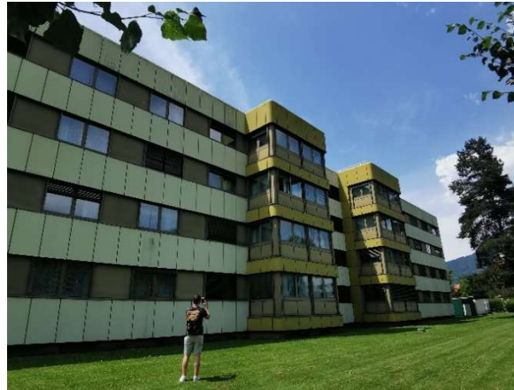
Figure 46: Pilot project Knittelfeld before renovation© AEE INTEC
