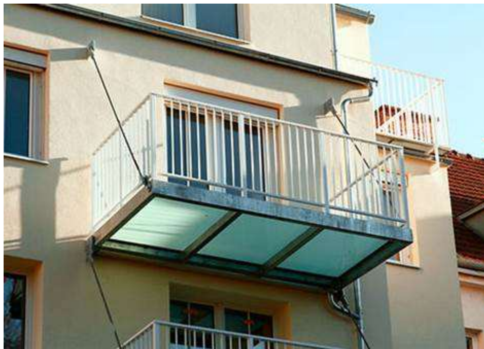
Figure 67: Single Construction Close-up Site Wattmannngasse 24, 1130 Vienna, © Rhomberg
