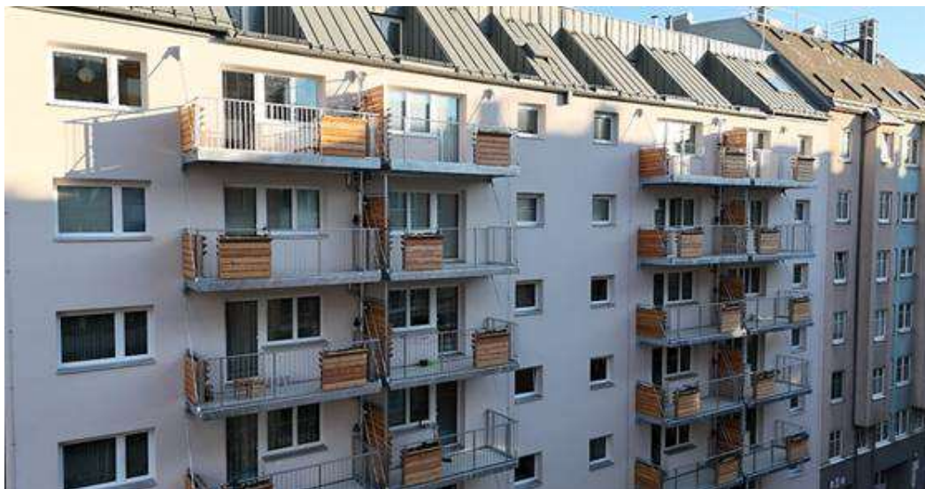
Figure 70: Completed Construction Site ESSBAR demo object, Karmarschgasse 59, 1100 Vienna, © Rhomberg
