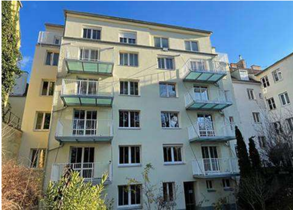
Figure 68: Completed Construction Site Wattmannngasse 24, 1130 Vienna, © Rhomberg
