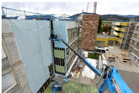
Figure 47: Construction Site Pilot Knittelfeld © Klimafond/Krobath
