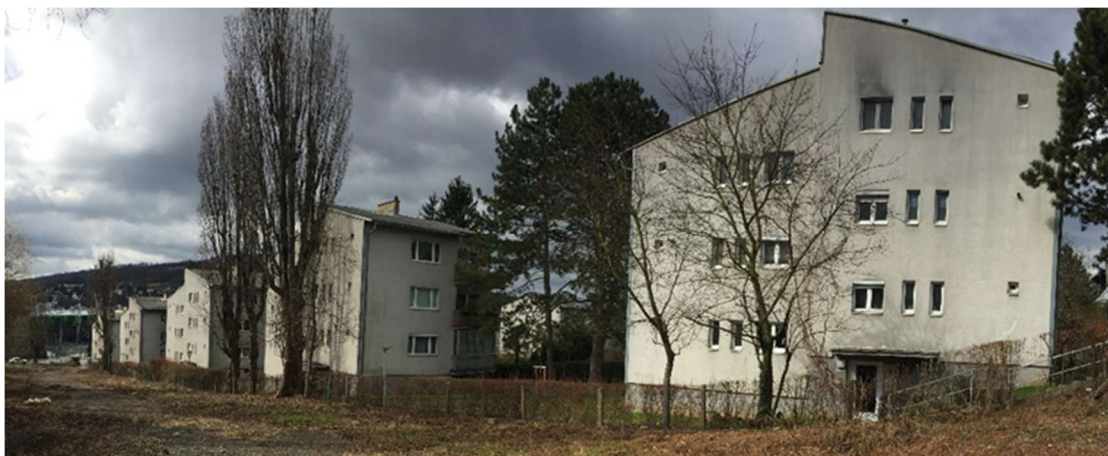
Figure 51: Pilot project Linzer Straße (© AEE INTEC)
