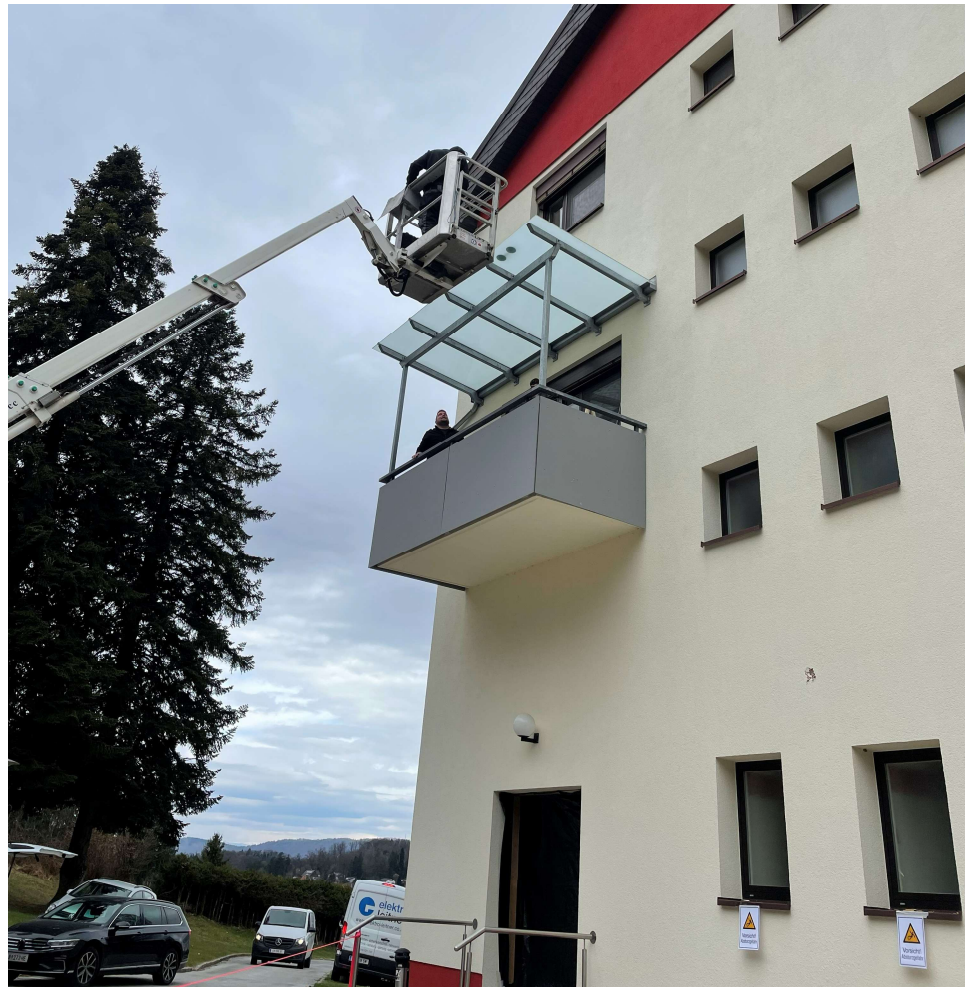
Figure 66: Deconstruction of a glass canopy © BauKarussell
