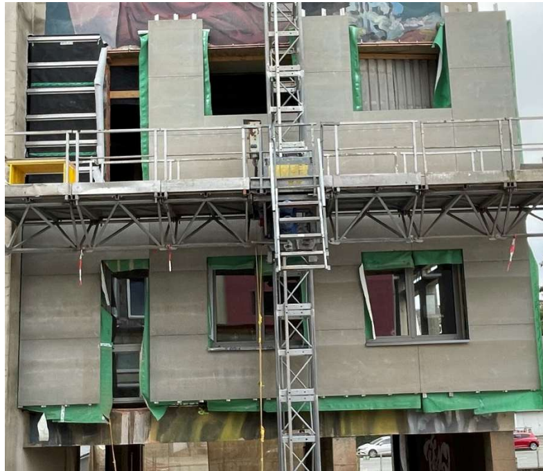
Figure 72: First façade elements are already on the wall © AEE INTEC
