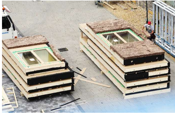
Figure 48: Prefabricated façade modules delivered on site © Klimafond/Krobath
