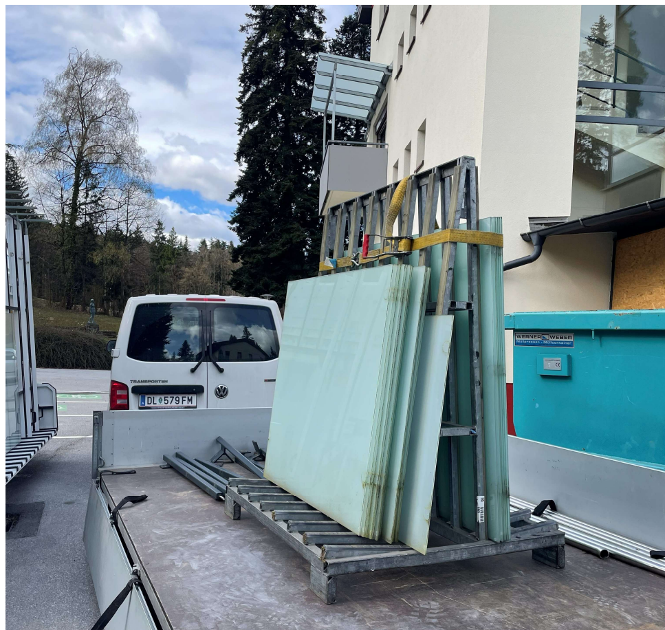
Figure 65: Glas elements prepared for transport to the new location © BauKarussell
