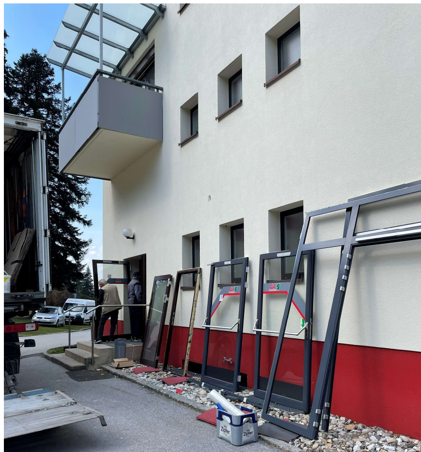
Figure 63: Dismantled door frame components ready for pick up © Baukarussell
