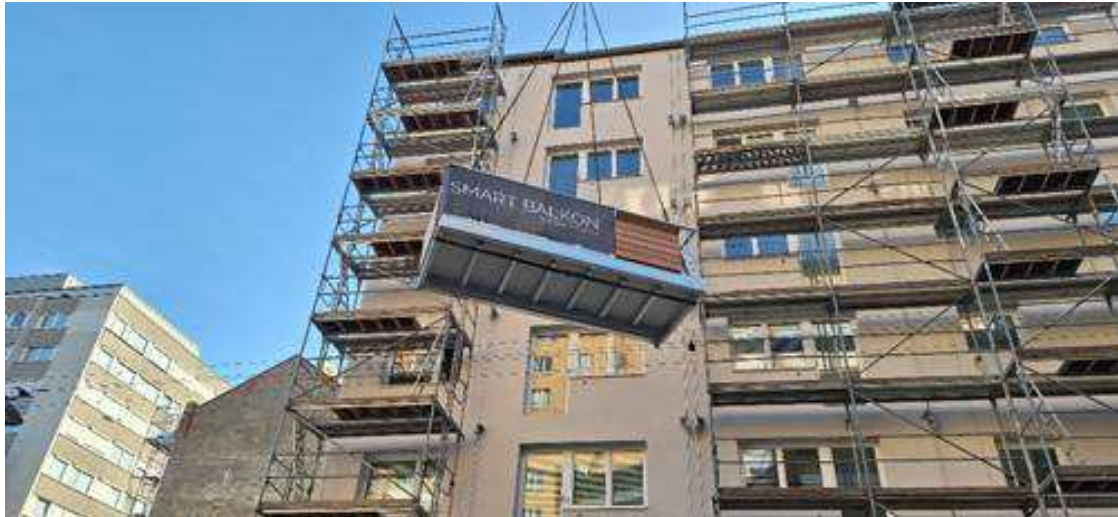
Figure 69: Work in Progress: Construction Site ESSBAR demo object, Karmarschgasse 59, 1100 Vienna, © Rhomberg
