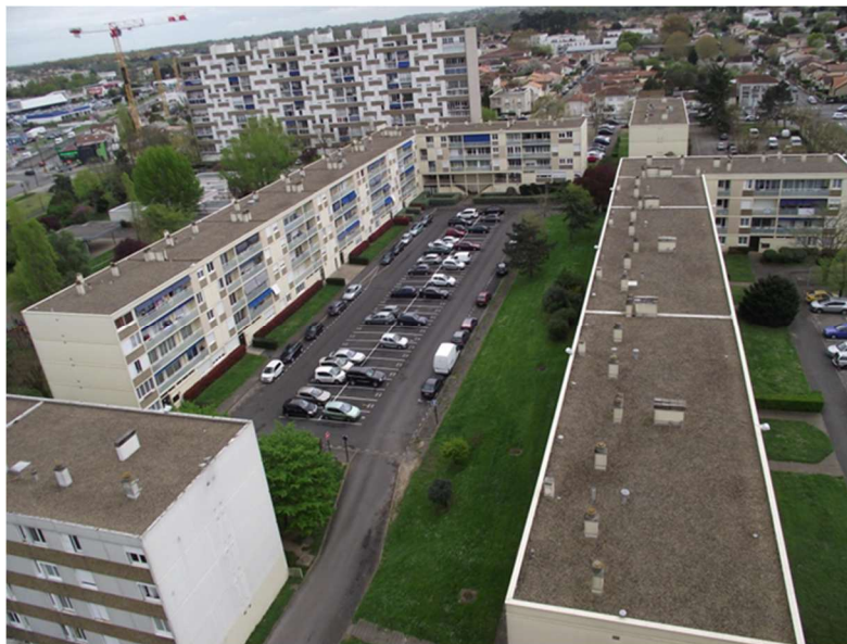
Figure 78: View of the Palm P, the French pilot project, before renovation ; @DomoFrance
